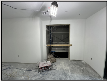
Elevator in Entryway
