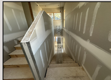
Staircase Between Floors
