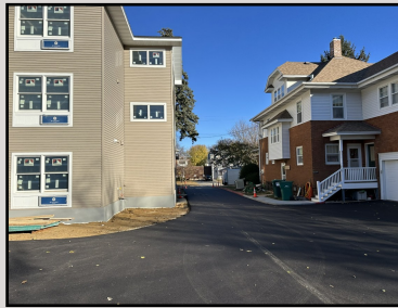
Parking Lot Entrance
