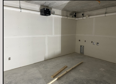
Basement Laundry Room
